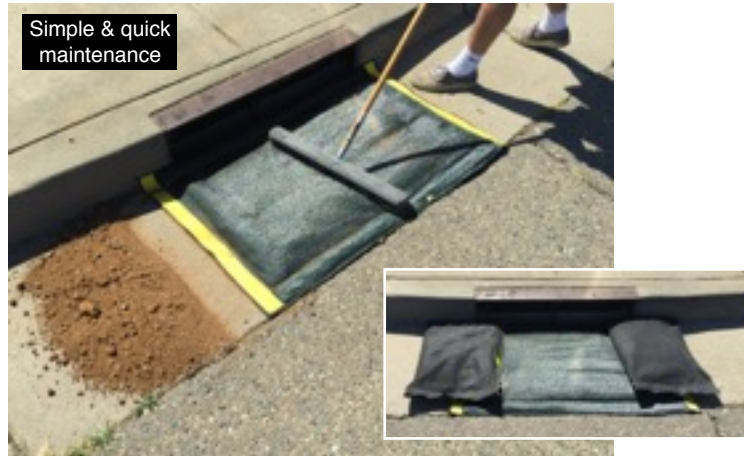
Step 2 Filter bottom
